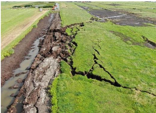
Figure 1. Recent failure of a dyke founded on organic soils
