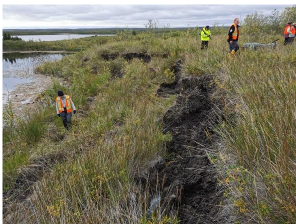
Figure 1: Collapse of the DMS clay cap at Tuk L-09.
