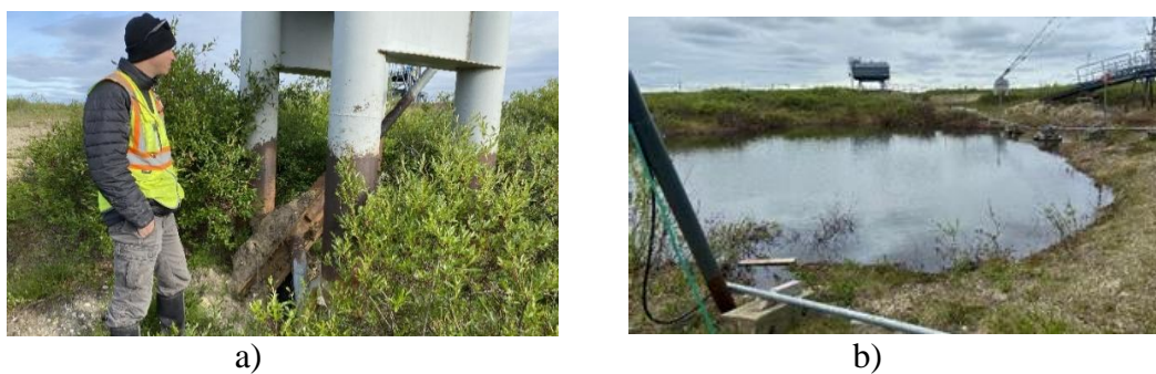
Figure 1: a) Effects of ground subsidence on piles and b) Thermokarst pond at a radar site near Inuvik, Canada
